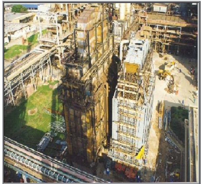
NEW HEATER MOVING PHASES – SARAS, Sarroch Refinery - ITALY
