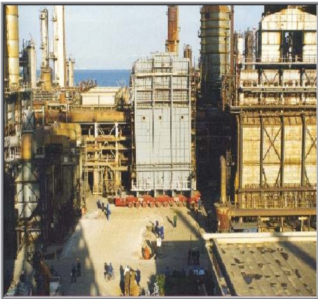
NEW HEATER MOVING PHASES – SARAS, Sarroch Refinery - ITALY
